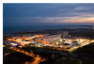
Shidao Bay HTR-PM Demonstration Project
