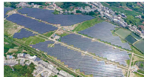
Tongshan Nanlin Flexible Bracket PV Project
