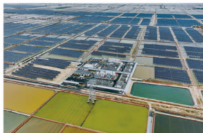
Shanyan Solar PV Plant
