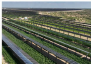
The Mengjiawan Photovoltaic Project
