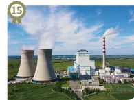
15 China Huaneng Group Co., Ltd. Jilin Branch Cogeneration (by Dong Chang)
