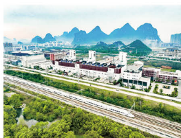
Huaneng Guilin Gas Distributed Energy Co. Ltd.
