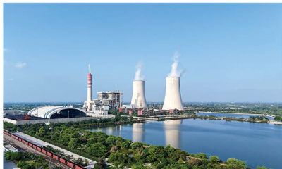
The Sahiwal Power Plant
