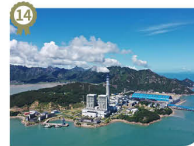
14 China Huaneng Group Co., Ltd. Fujian Branch Luoyuan Power Plant (by Jia Hongjiang)
