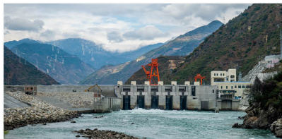
Sichuan Yingliangbao Hydropower Station
